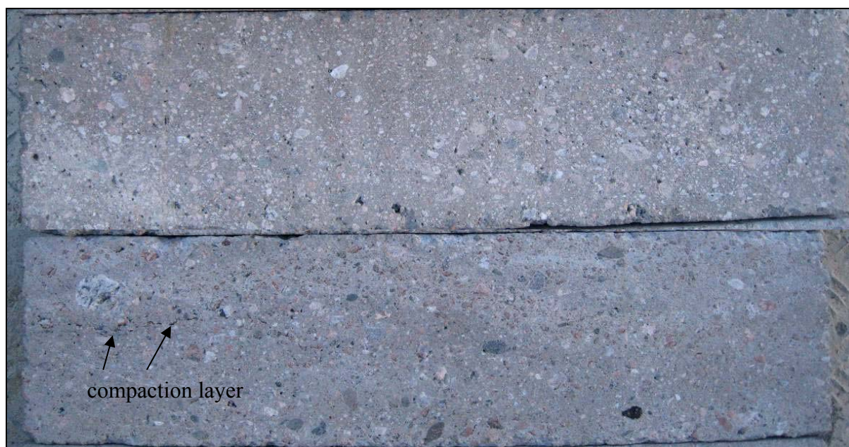
PICTURE 1. The inhomogeneous shotcrete shown here in the shrinkage prisms. The reference at top, the T25 prism at bottom.
